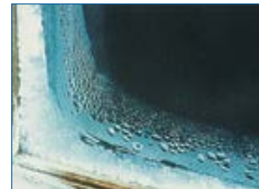
Window condensation can fuel mold growth.
